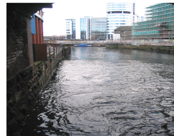
Dark Arches, Granary Wharfe
